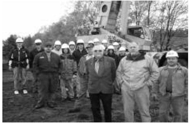
Vilas Machmueller, EMPD Chief Dan Vergin, DCE Construction Teacher Chad Pernsteiner stand with members of the Village Crew that tore down the Steppert home and DCE High School students who built the new Habitat for Humanity home.
